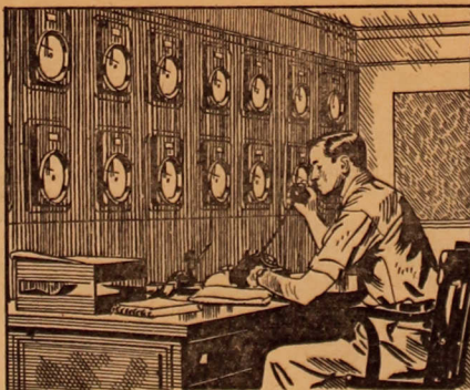
Measuring Stations Miles Apart Are Monitored in This Room
