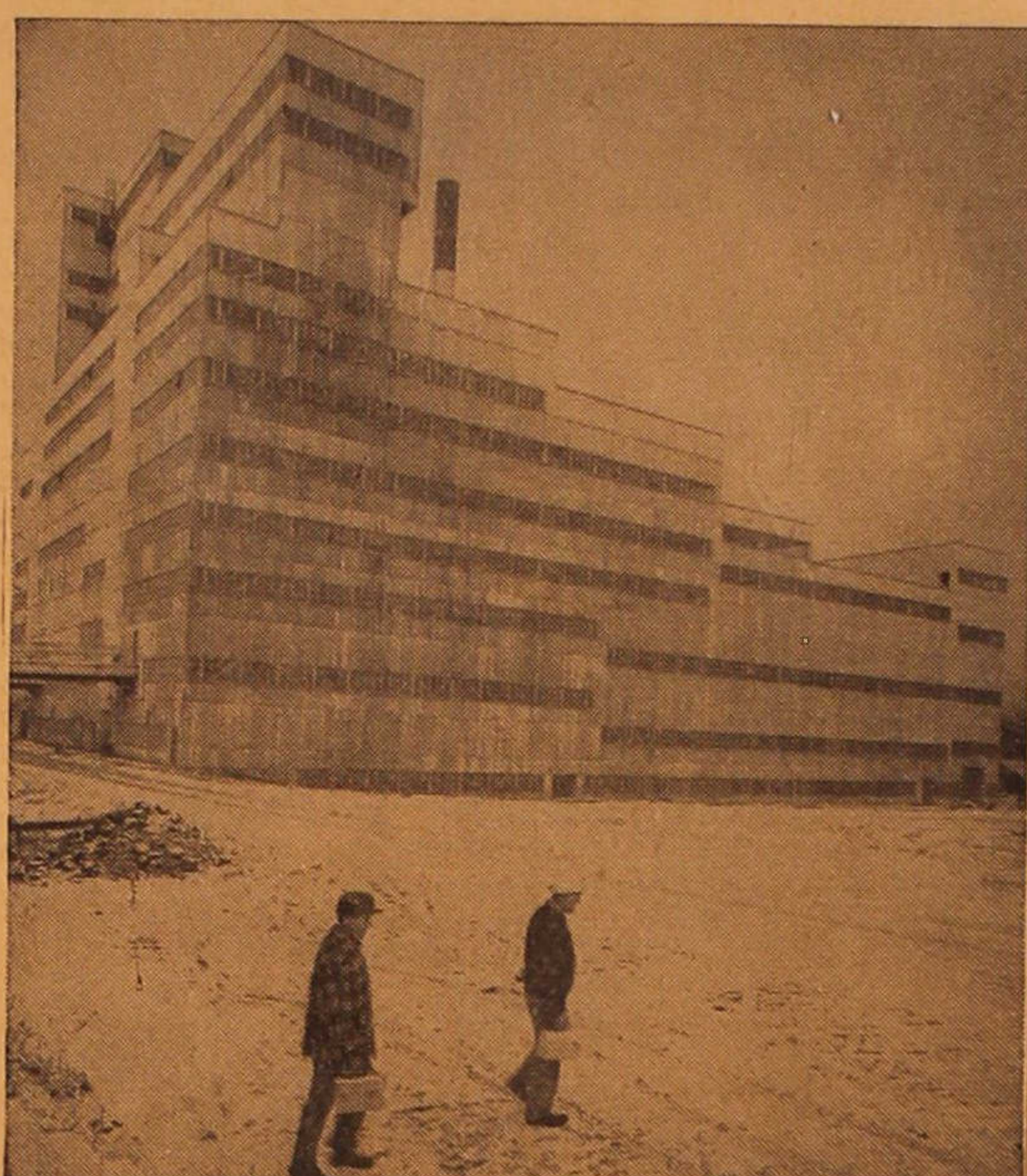
This ten-story addition to U. S. Steel's Frick District's Robena coal preparation plant was placed in operation the early part of 1954. The plant is now washing 23,700 tons of coal, the entire daily output of the Robena Mine. In the foreground are Thomas McKeeny, left, and Rudolf "Red" Ingram, fine coal second helper operators at the plant.
