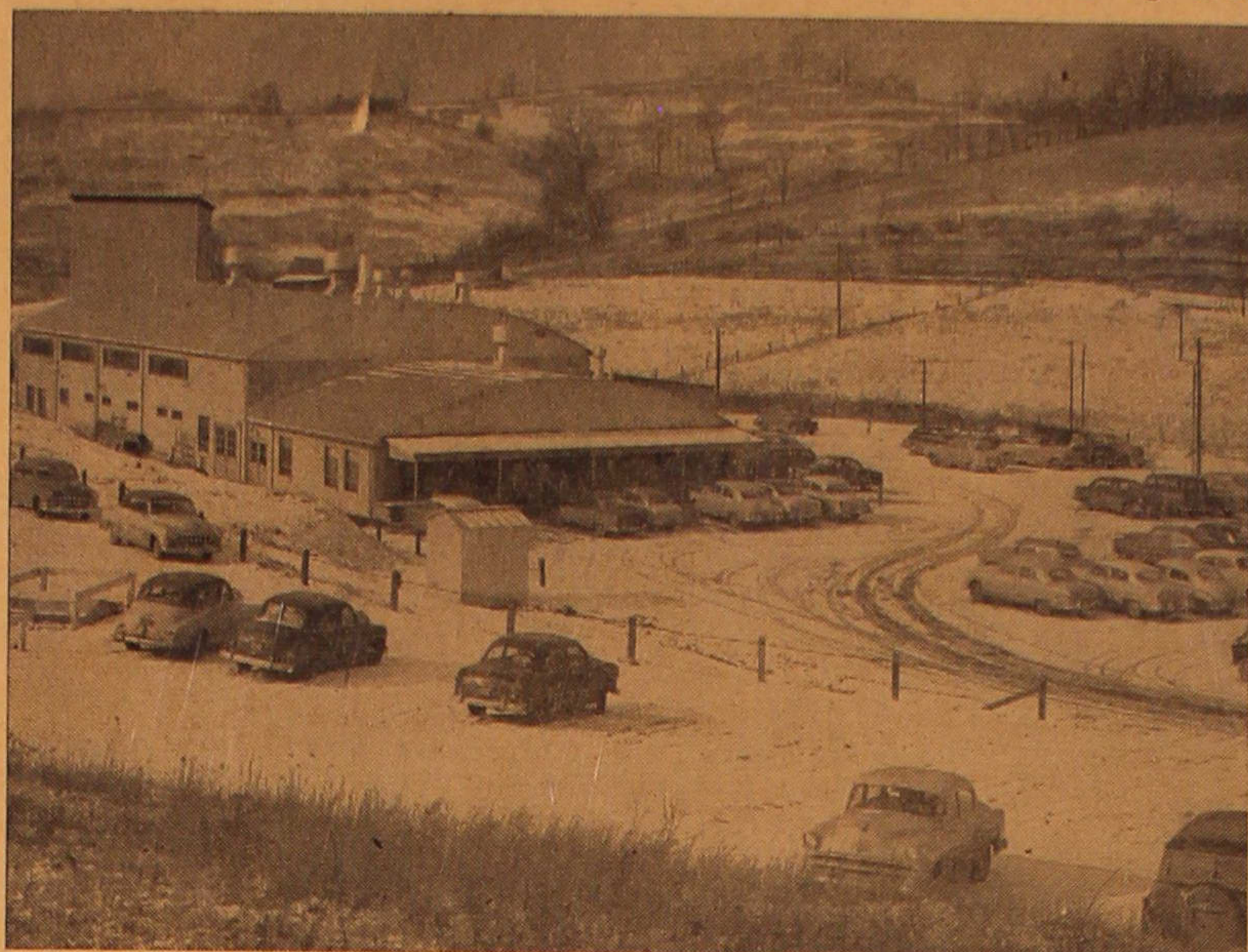
New service facilities at U. S. Steel's Frick District's Bowlby Shaft, located in Cumberland Township, was placed in operation in 1954. The 558-foot shaft is used daily by about 870 miners.
