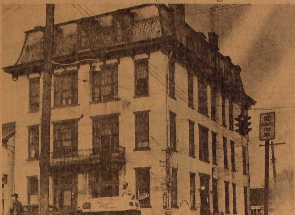
The Walton Hotel, which stood for many years at the northwestern corner of High and Morris Streets in Waynesburg (now a public parking lot) was one of the many hotels which flourished in Greene County before automobiles removed most of the need for their existence which is discussed in today's "Fact and Folklore" column on this page.
