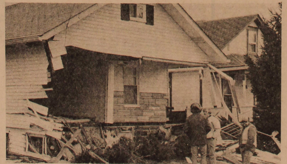
Some of the damage caused to the Mrs. Mary Matyk home
