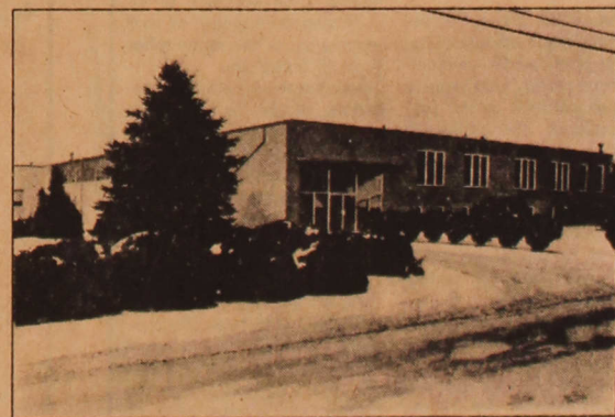
With county support, Leder, Inc. moved into this building at Carmichaels during the past year.
