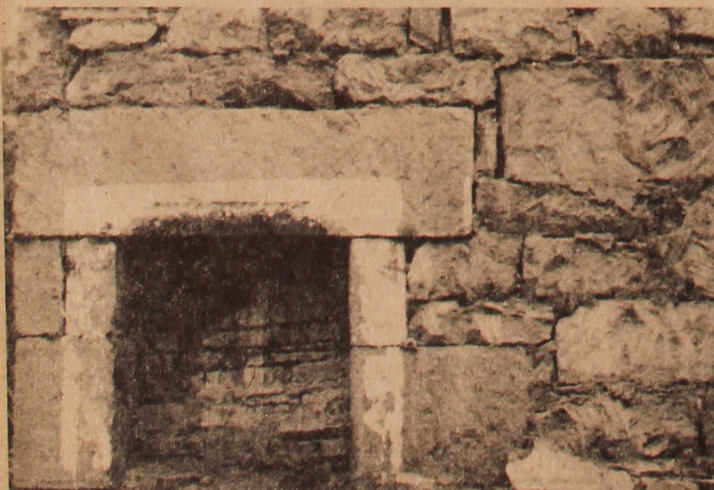
Cut-stone fireplace from the original log cabin will be preserved.
