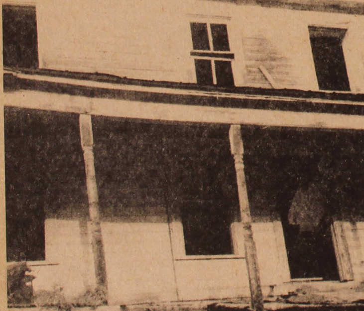
Siding, and additions, conceal original log cabin.
