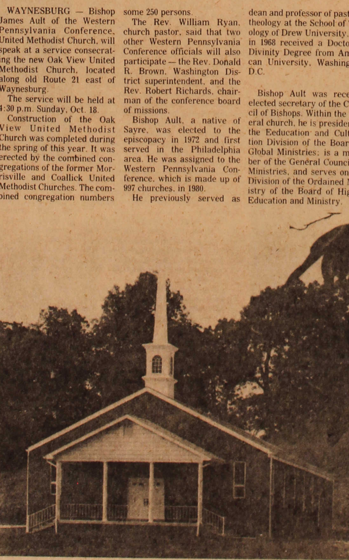
Oak View United Methodist Church, which was built this spring.
