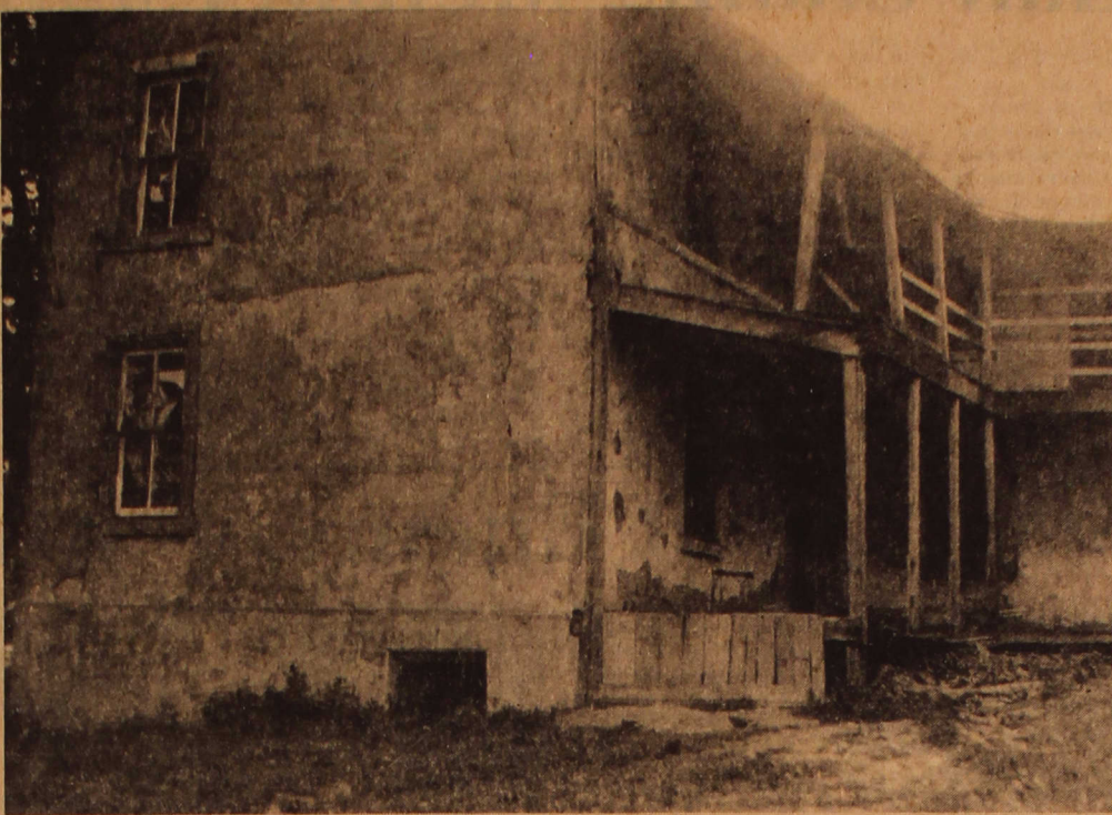
Pictured is the last stages of the one-time palatial Buchanan homestead which stood on the high bluff above Route 21 in West Waynesburg, about a half-mile west of the Waynesburg borough line. The owner and builder of the once sturdy stone structure was Attorney A.J.A. Buchanan, a native of eastern Pennsylvania who became ill with a fever while traveling to Kentucky to practice law. As he regained strength, he decided to remain in Waynesburg and founded the law firm of Buchanan and Walton. He lived in Waynesburg until his death. The property on which the home stood is now a mobile home court owned by Mrs. Anthony Gusic.
