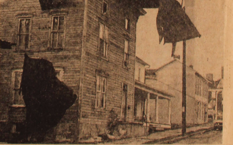
Observer-Reporter Photo Wind Damage More than 1,770 Waynesburg residents were left without electricity when high winds Monday peeled the tin roof from this house on South Washington Street, dropping it across West Penn Power Co. lines. The house, owned by Farley Toothman, is occupied by Steve Samuels. This picture shows a large section of the roof as it falls from the side of the house while another section of roof hangs over a power line.
