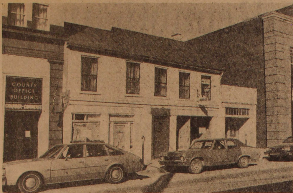
Sayers-Hooper building on High Street in Waynesburg
