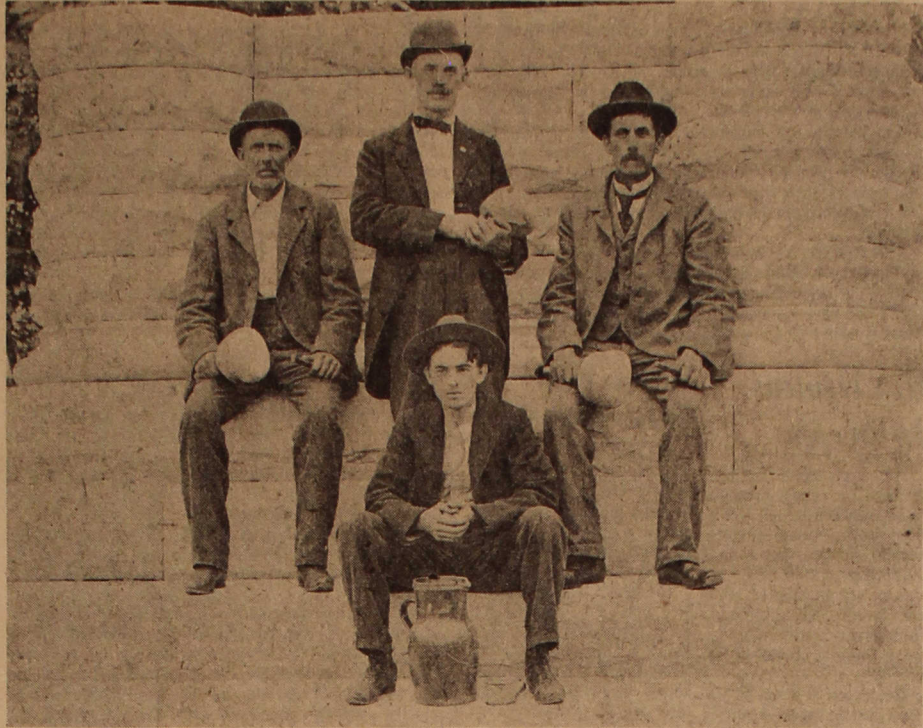
The unidentified stone masons were working on the Soldiers' and Sailors' Monument in the Waynesburg park. The monument was erected by S.A. Rinehart whose other projects included the residences of J.B.F. Rinehart, Dr. J.T. Ullom and C.W. Bowlby and the First Christian Church. Rinehart's marble and granite works were located on South Morgan Street.
