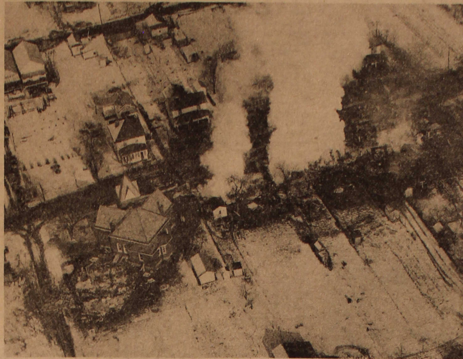
This was the scene in Jefferson on Feb. 9, 1951, shortly after three separate sewer gas explosions demolished six homes killing two and injuring eight.
