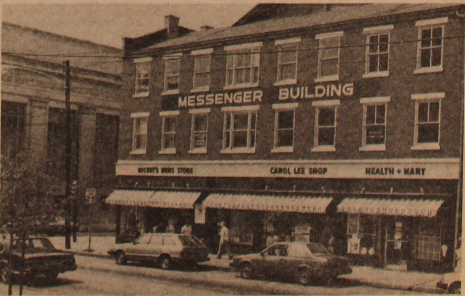
This is the Messenger Building following renovation under the WECR project.
