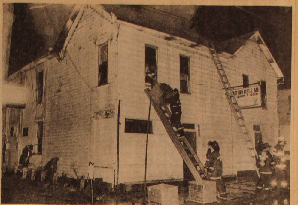
Firemen battle blaze which destroyed East End Restaurant
