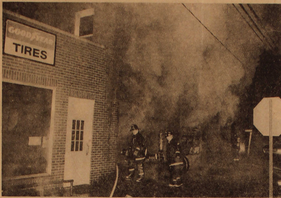
Smoke pours from the Waynesburg Auto Center building during a fire early Monday.
