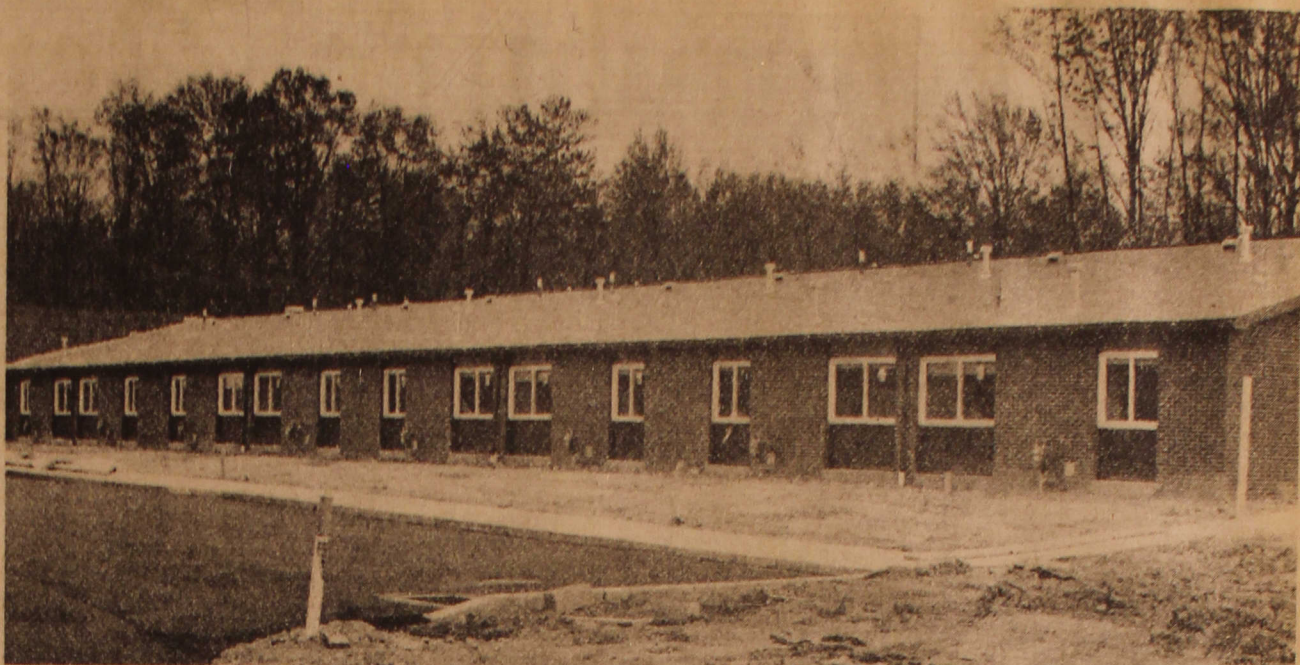
Apartment building for the elderly in Carmichaels nearing completion
