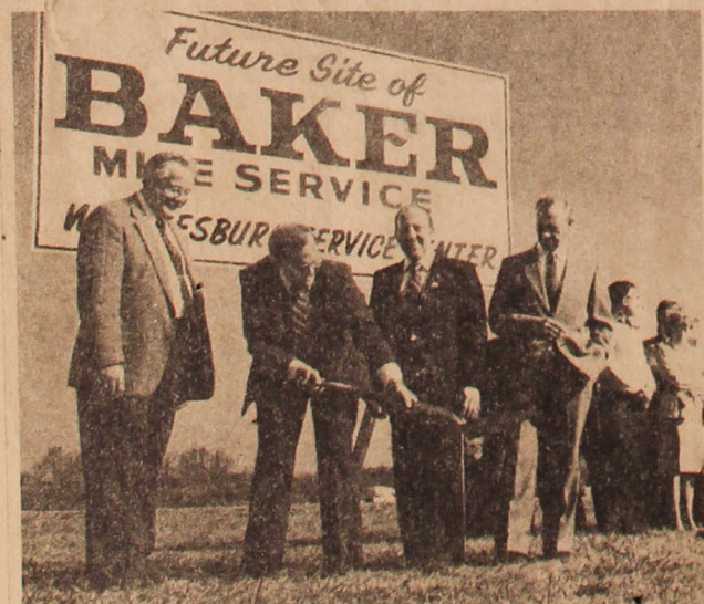
Ground broken on Oct. 30 for $3.5 million Baker Mine Service building near Waynesburg
