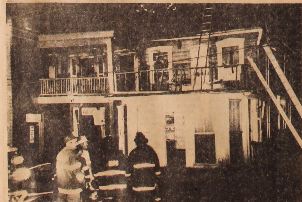
Waynesburg firemen battle apartment house fire at Greene and Morgan streets.
