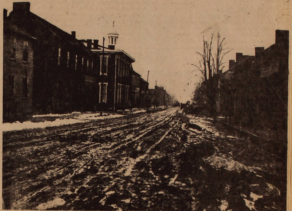
This was High Street in Waynesburg looking west sometime near the turn of the century. Most of the buildings have since been razed.
