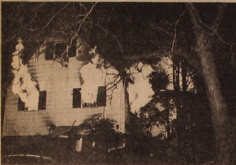
Flames burst from T. William Barnes home in Franklin Township.
