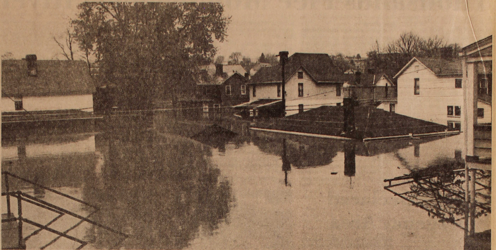
Floodwater reaches some rooftops in West Brownsville.
